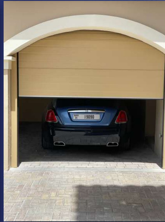
Garage Shatter Task: Design and Build Location: Dubai, The villa
